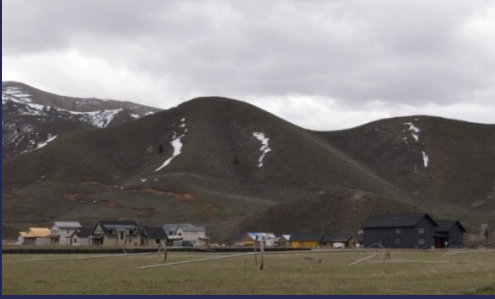
Photo Caption: The Quigley Farm development currently under construction in Hailey, Idaho blends for-profit and nonprofit models in an effort to provide both purchase and rental affordable housing options.
